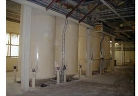
Photo 2. The silos for the interim storage of incoming raw materials.
