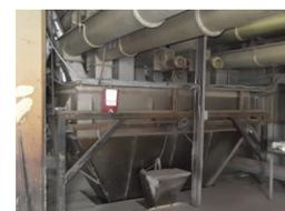
Photo 5. The weighing system for the small solid components.
