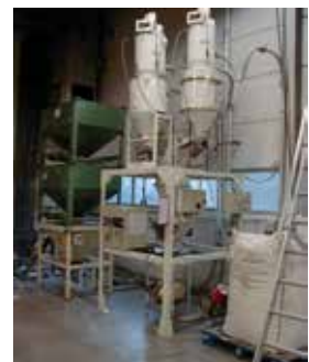
Two hopper system for a continuous flow
