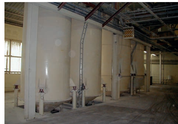
Fig. 2 Weighing silos for loading the compartments of bulk trucks
