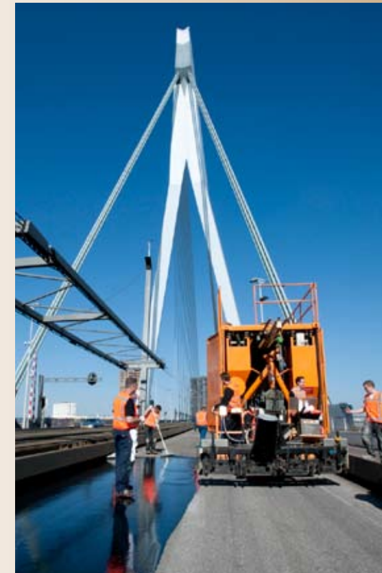
applying the wear layer on the Erasmusbridge.
