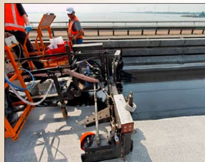
applying the layer on the Moerdijkbridge.
