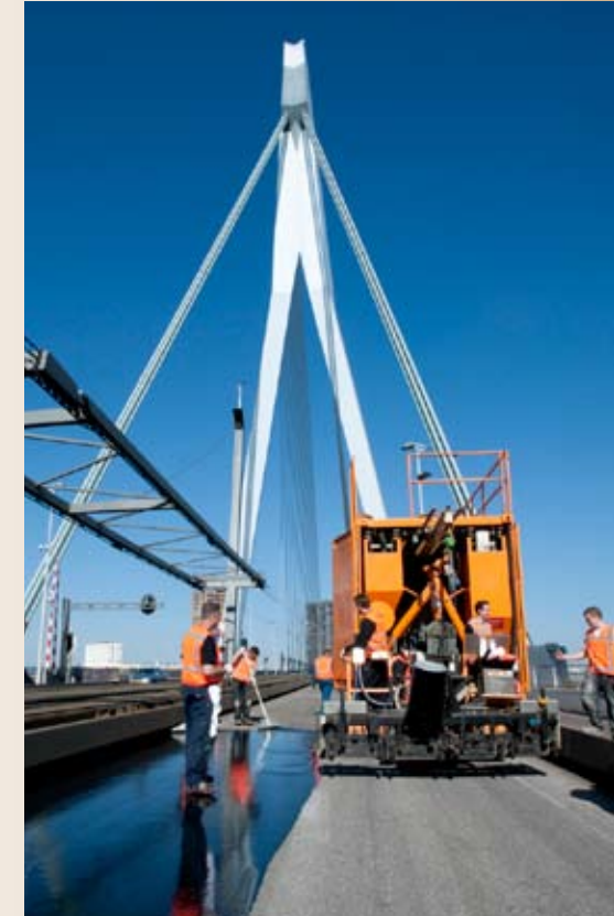
applying the wear layer on the Erasmusbridge.
